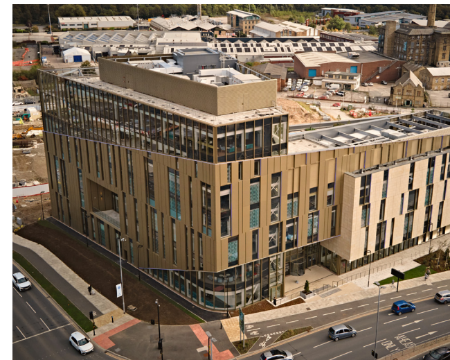
The Daphne Steele Building at the National Health Innovation Campus in Huddersfield
